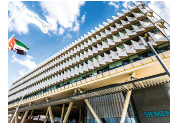
Siemens Middle East HQ at Masdar City
