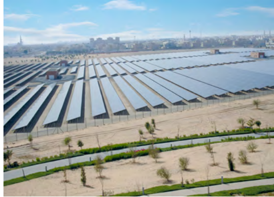
10 MW Solar Farm
